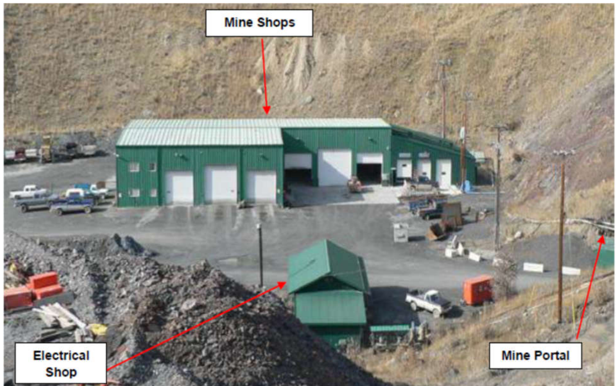
Figure 6-2. Existing BRM infrastructure; mine portal area.
